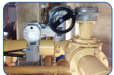
Plug Valve in Sewage Treatment Plant
