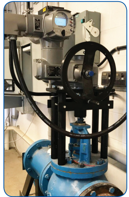
Globe valve Ottawa pump station
